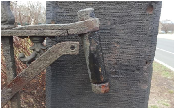
One of three gates with rusted, frozen, and broken hinges—Top and bottom hinge illustrated.
