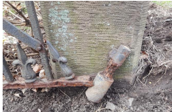
One of three gates with rusted, frozen, and broken hinges—Top and bottom hinge illustrated.
